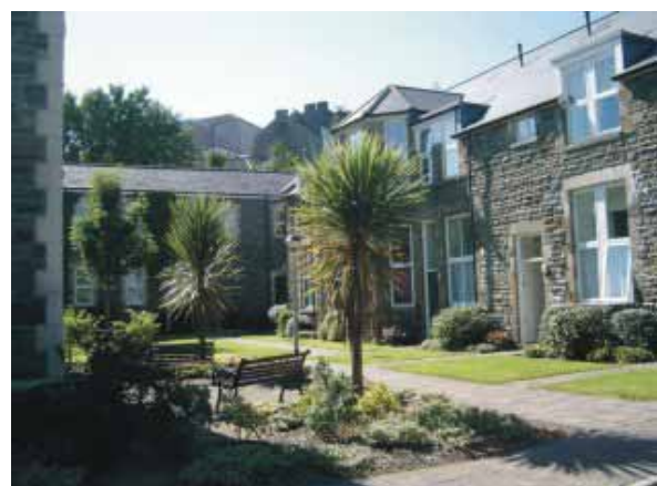
Urban Regeneration, The Courtyard, Old Hospital, Swansea
